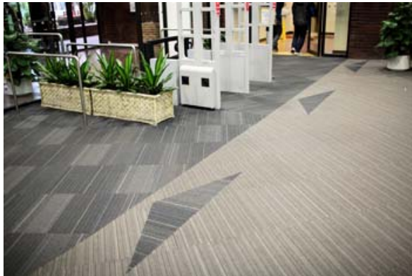
Carpeting in a contrasting color and pattern have been installed to bring attention to the inclines of the raised flooring
